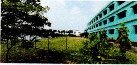
School Building and Playground
